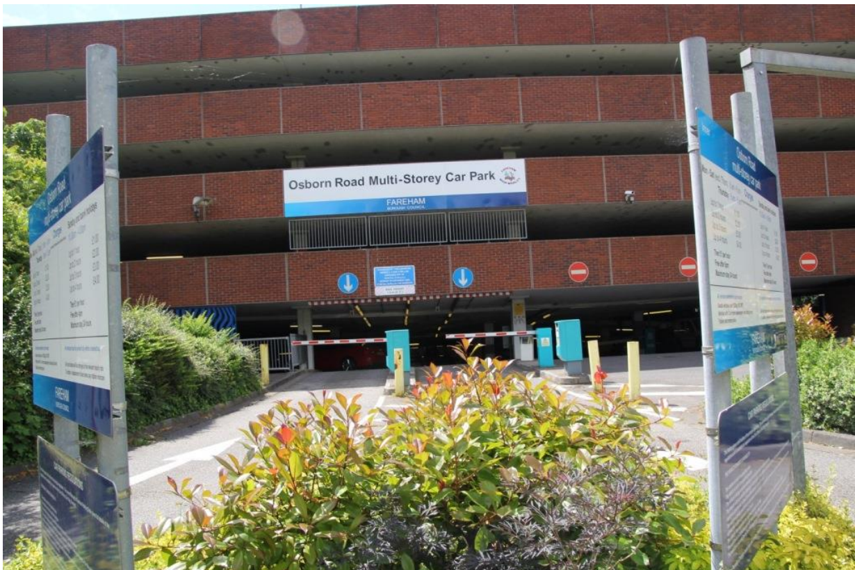
Osborn Road Multi-Story Car Park
